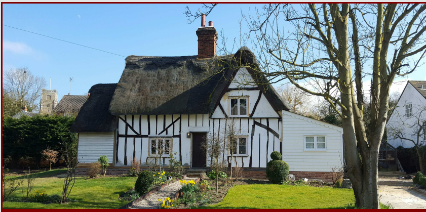
The black and white timber framed house in Thaxted is called Dick Turpin's Cottage but was probably in fact premises used as a butchers shop.
